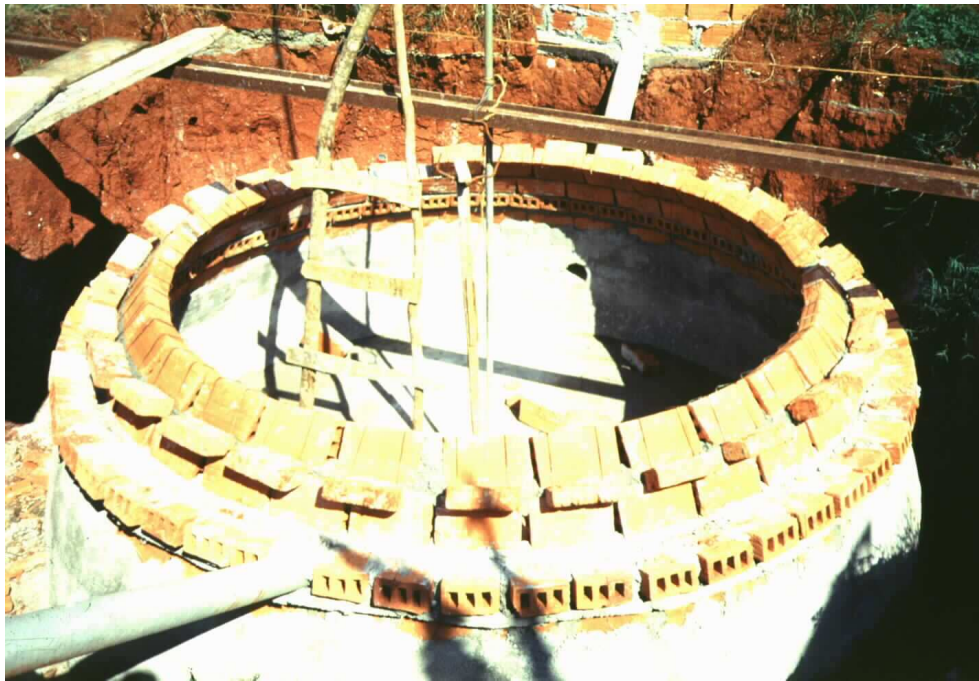
Above: Fixed dome biogas fermentation chamber under construction
