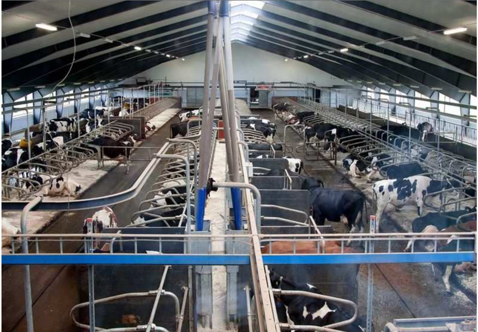
Loose box cow shed with mechanical dung removal
